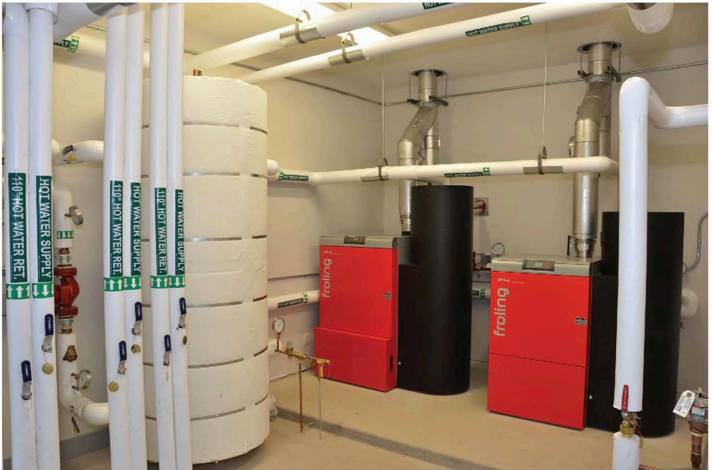
The boilers share a main mechanical room with a super-insulated, 400-gallon buffer tank. All supply and return lines to both buildings run underground.
